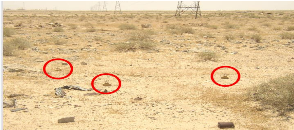
Mines spread near electric power transmission towers
